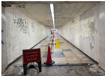
Work begins on the subway transformation
